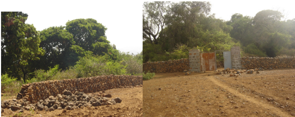
Fig 5. Typical Stone wall
