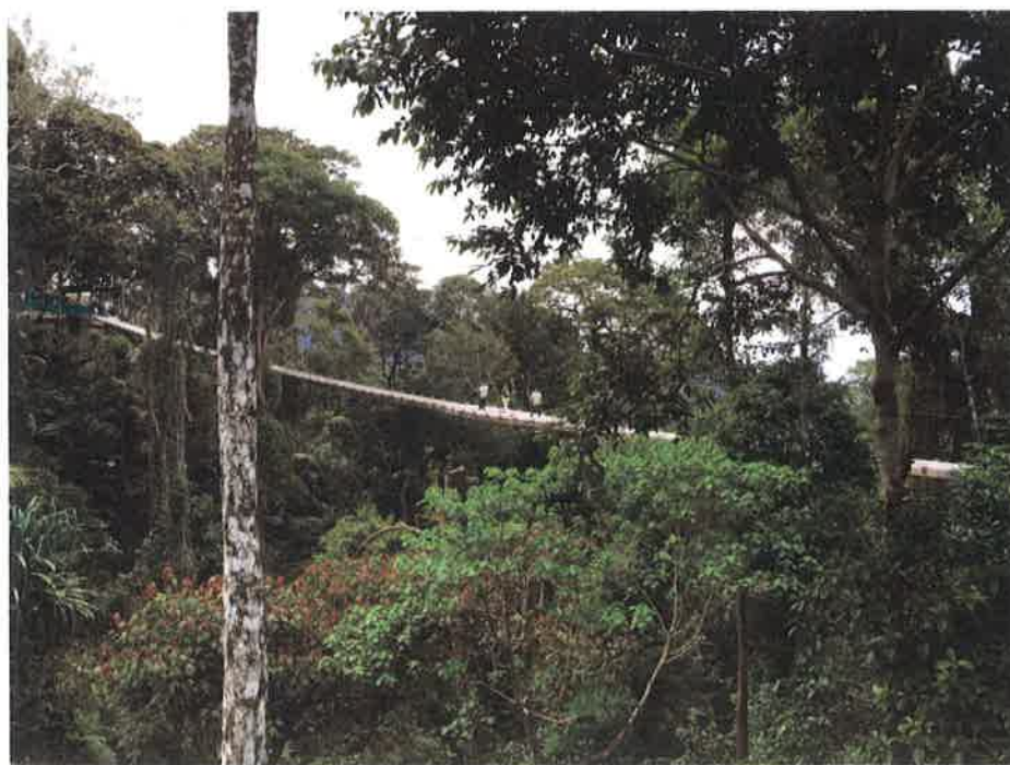
Canopy walkways are complete on Penang Hill, Malaysia
