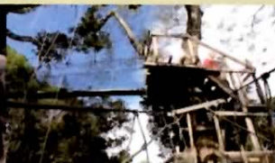
WALKWAYS OF THE WORLD - ACTS Canopy Walkway, Peru
