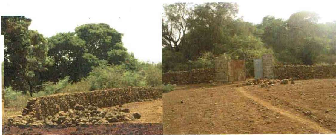
Fig 5. Typical Stone wall
