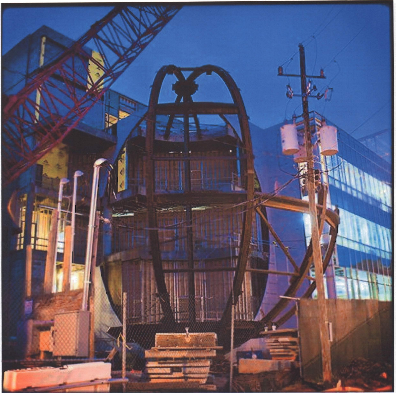
March 11 - Construction of The Daily Planet Technology Theater at The Nature Research Center, Raleigh NC.
